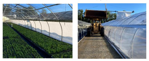
**Figure 12.** (left) A 9x44 m (30x145 ft) greenhouse covered with 50% shade cloth and 2 m (6-ft) plastic side curtains. (right) Applying a double layer of clear plastic to greenhouse using boom attachment.
