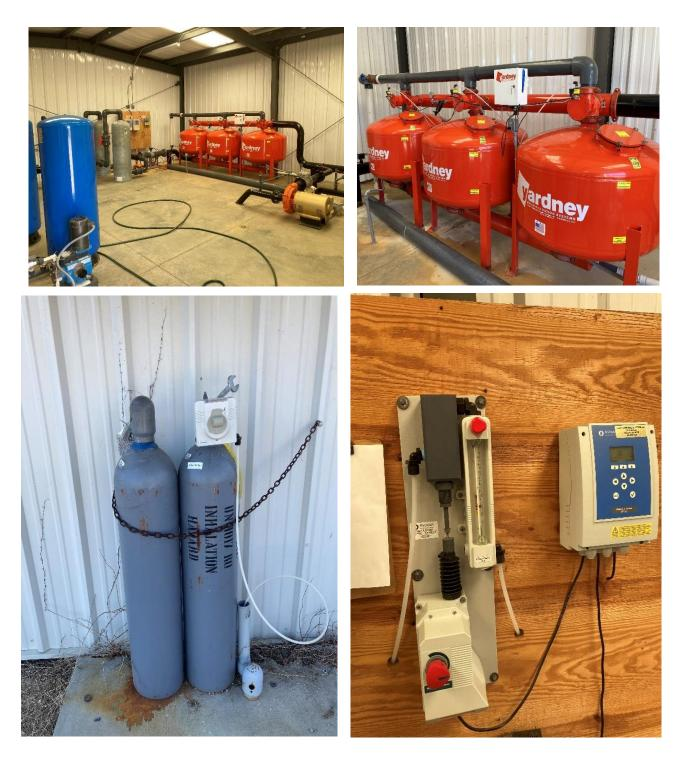
**Figure 17.** (top left) Interior view of pump house, (top right) a Yardney sand filtration system with automatic backflush, (bottom left) chlorine gas cylinders with a regulator, and (bottom right) a Wallace and Tiernan<sup>®</sup> S10k gas feed chlorine metering system.
