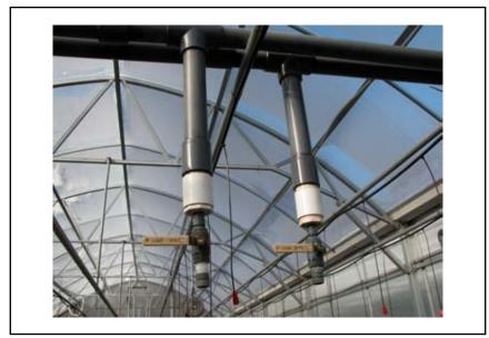
Figure 5. Schedule 80 PVC will not prevent algae growth inside irrigation lines.
