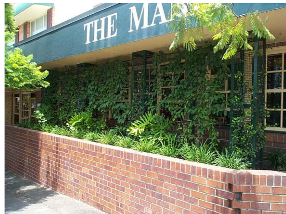
Figure 2. The structure at Manly Hotel in Brisbane has a west facing wall; the integration of a green façade helped to lower the indoor temperature by up to 5°C.
